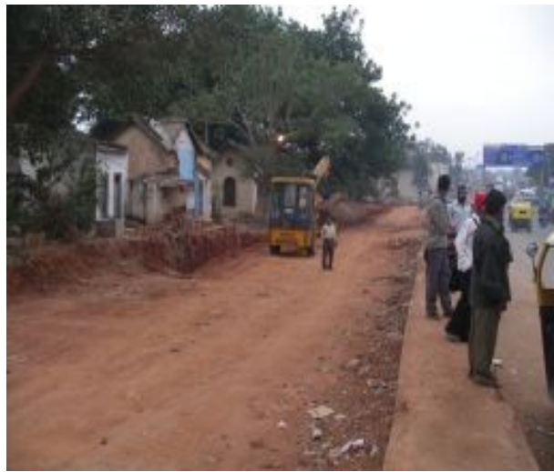
Bellary Road Widening- No heed pedestrians rights
