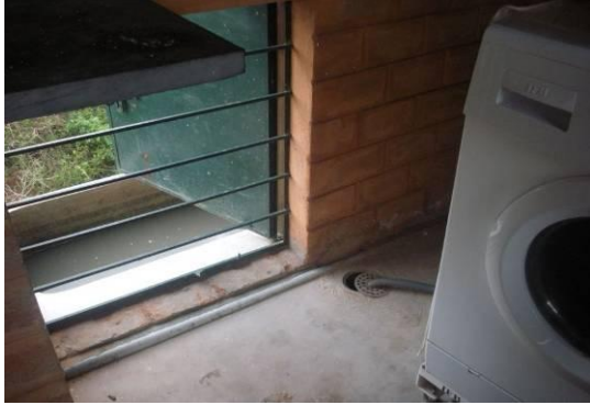
Picture 12 – Run-off from washing machine getting collected in the sump Picture 13 – Compost (Dry) Toilet
