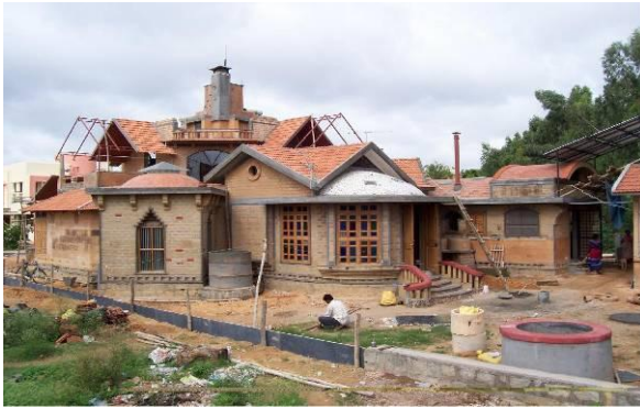
Picture 4 – Mr. Chockalingam’s house under construction
