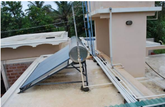
Picture 18 – Roof of the house coated with white colour paint reduces the amount of heat transmitted into the house.
